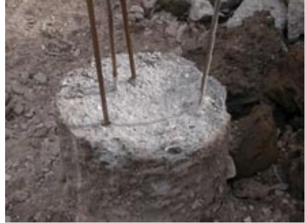
Good pile head preparation
