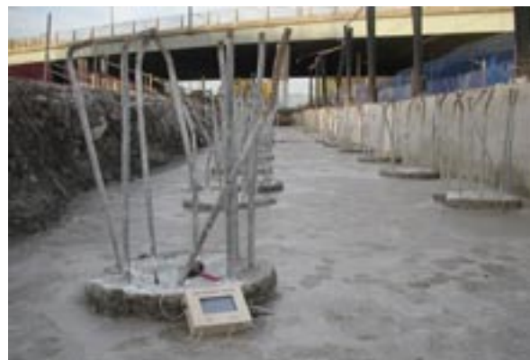
Good pile head preparation
