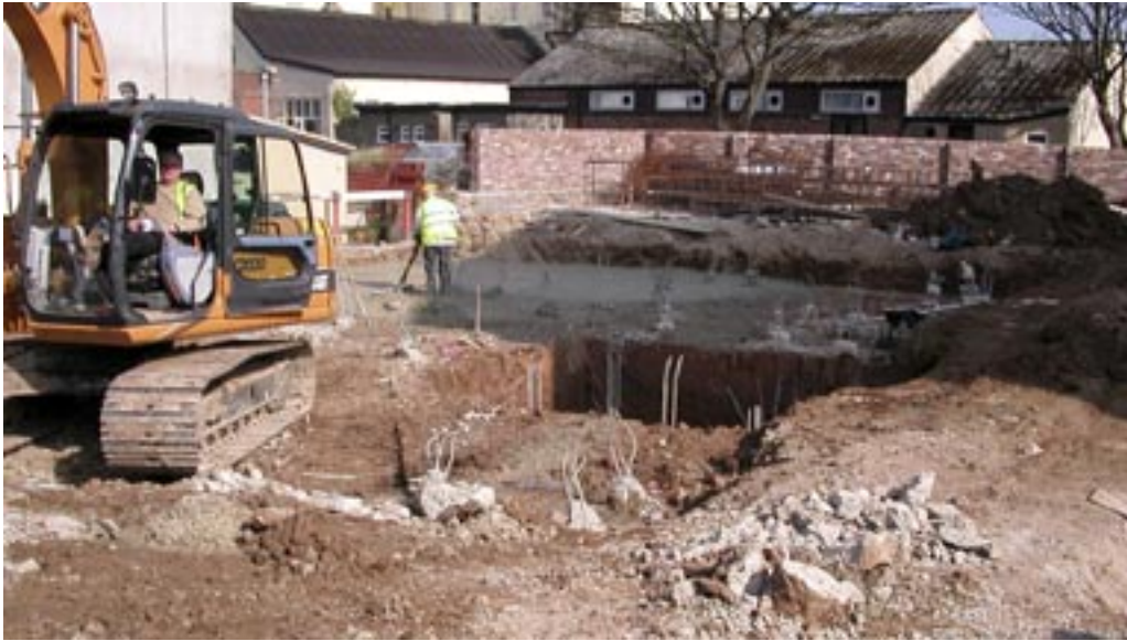
Poor site preparation for pile testing
