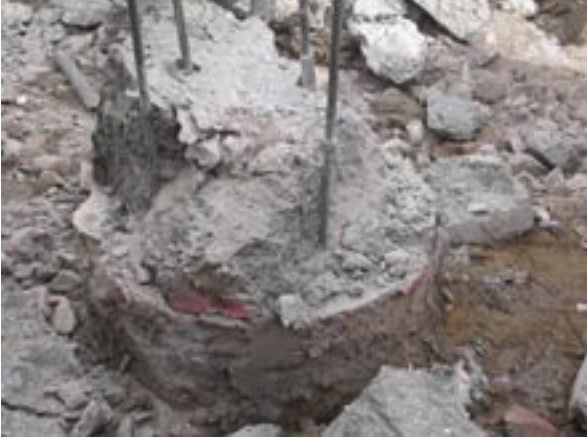
Poor pile head preparation
