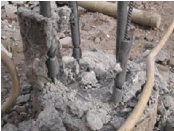
Poor pile head preparation
