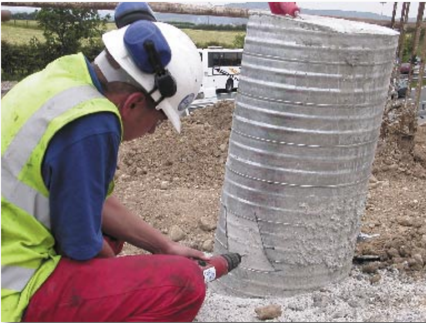
Bored pile head preparation
