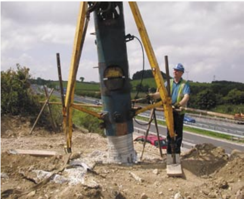
Inclined bored pile dynamic test
